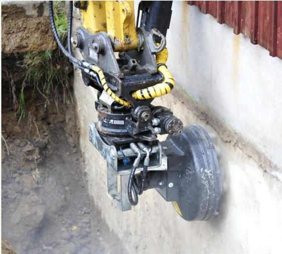
Milling of wall mounted on tiltrotator .
