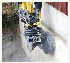
Milling of wall mounted on tiltrotator .
